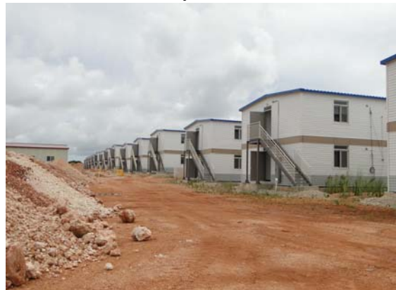
Image 2: Construction project in the northern part of the island.
