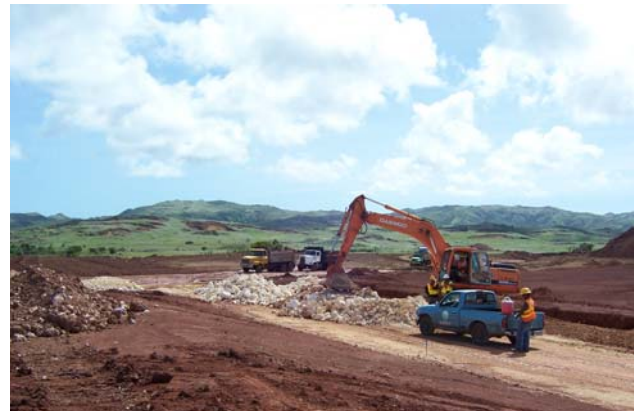
Image 5: Construction at the new landfill in Layon, Inarajan.
